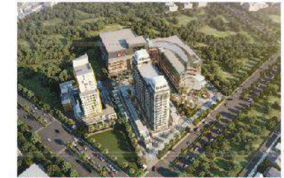
SECTOR 37 C, GURGAON-DWARKA EXPRESSWAY
